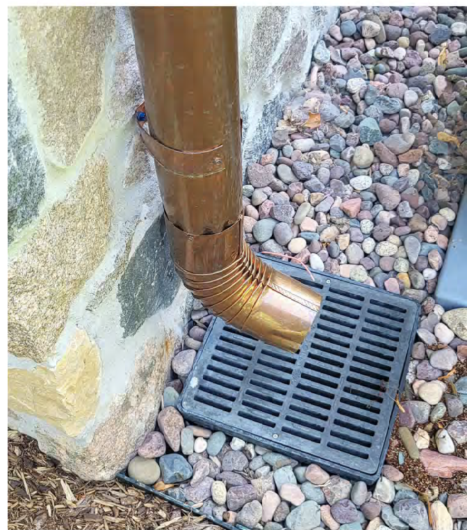
DOWNSPOUT TO DISCHARGE INTO 12" CATCH BASIN. TILE LINE TO DAYLIGHT AS GRADE ALLOWS IN GRAVEL APRON
